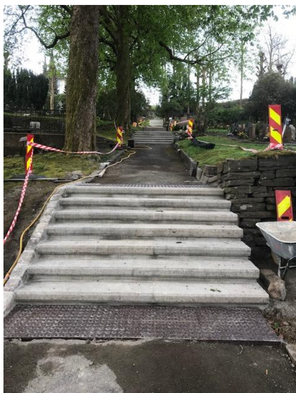
Møllendal - Trapp under rehabilitering
